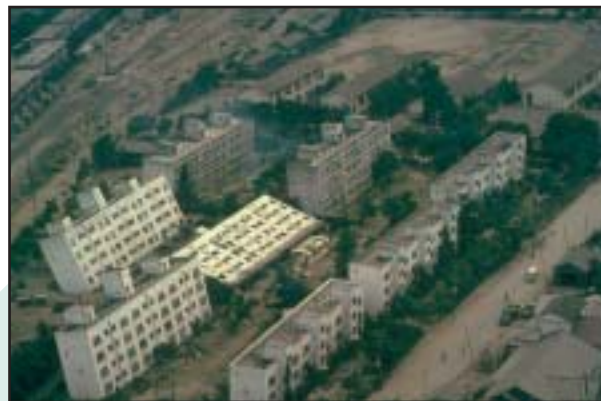
a) Bearing capacity failures of Kawagishi-cho apartment buildings
